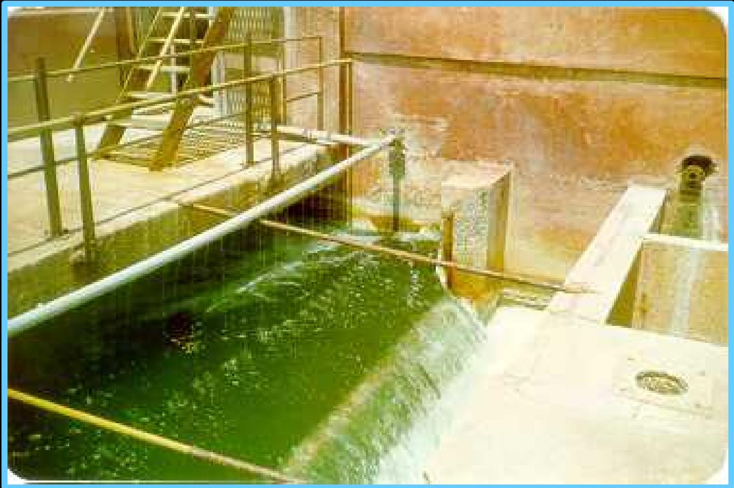
Chemical dosing through perforated pipe – Simple and effective
