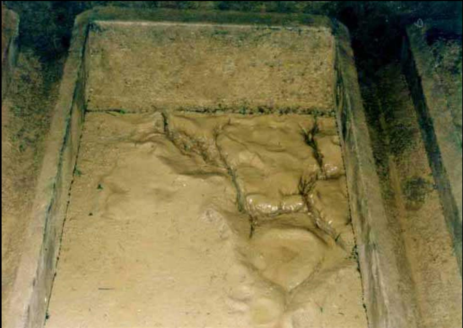
**Cracks in filter bed**
