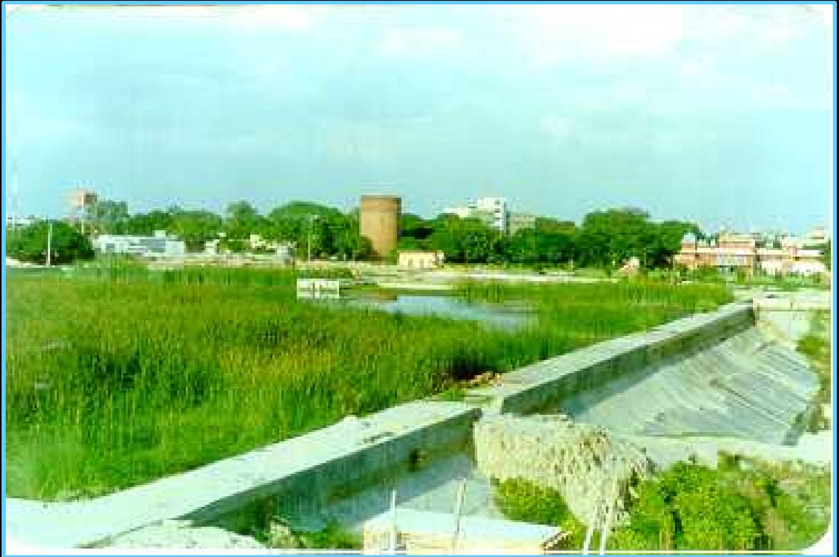
Silted sedimentation tank & aquatic weed growth
